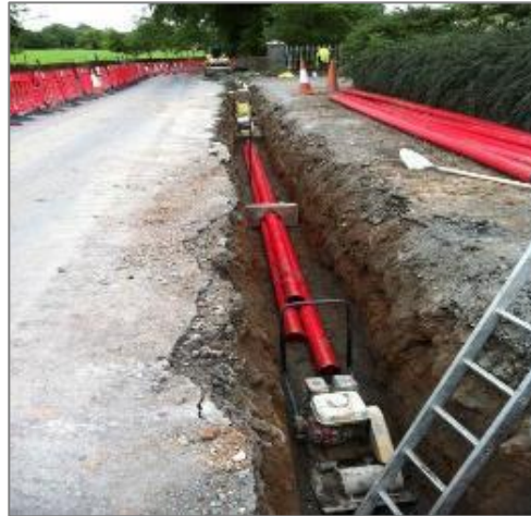
Figure 3 - 110kV Underground Duct Installation
