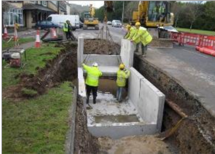
Figure 9 - Joint bay under construction (pre-cast)
