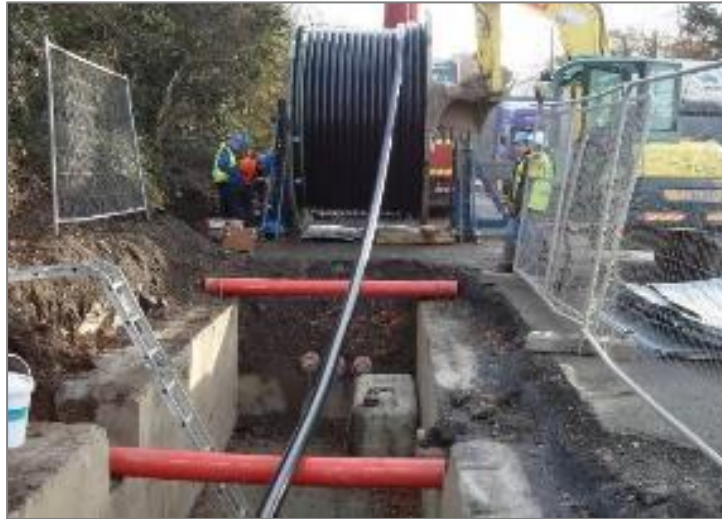
Figure 10 - HV cable pulling procedure (Typical drum set-up)
