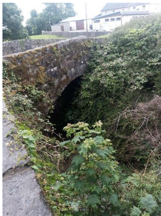
Figure 26 - Side view of Bridge 6 facing southeast.
